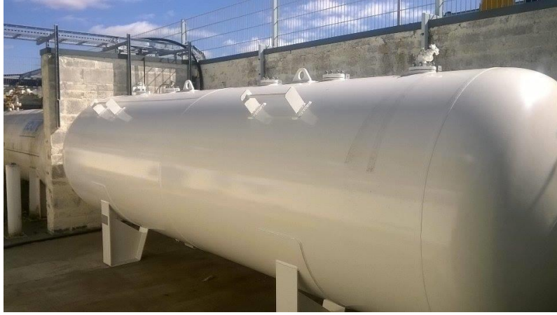
Figure 5-8: LCEP H 2 Tank. Courtesy of Bright Green Hydrogen
