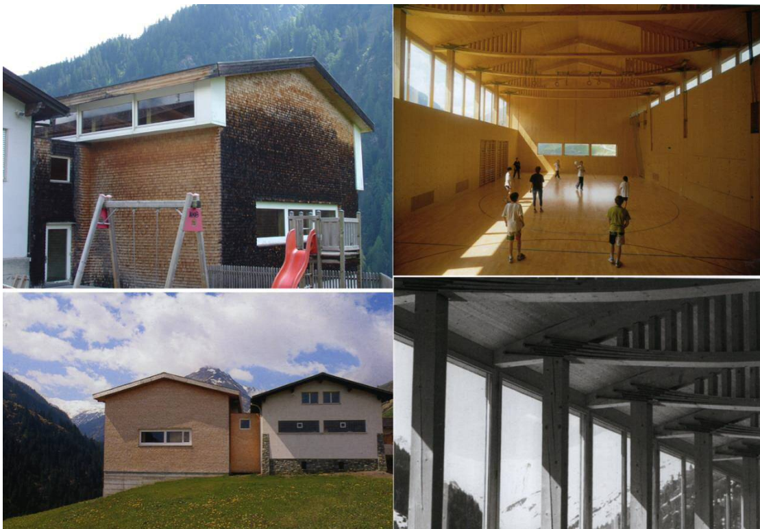
Figure 45: Sports hall. Upper left: exterior elevation; upper right: building interior; lower left: comparison with the old hall; lower right: window details
