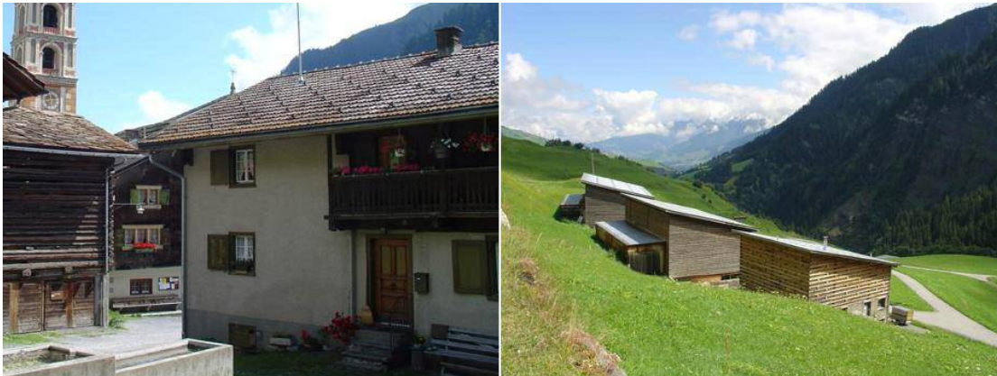
Figure 33: Buildings in Vrin. Left: building with contemporary materials; right: designed contemporary architecture with Strickbau concept
