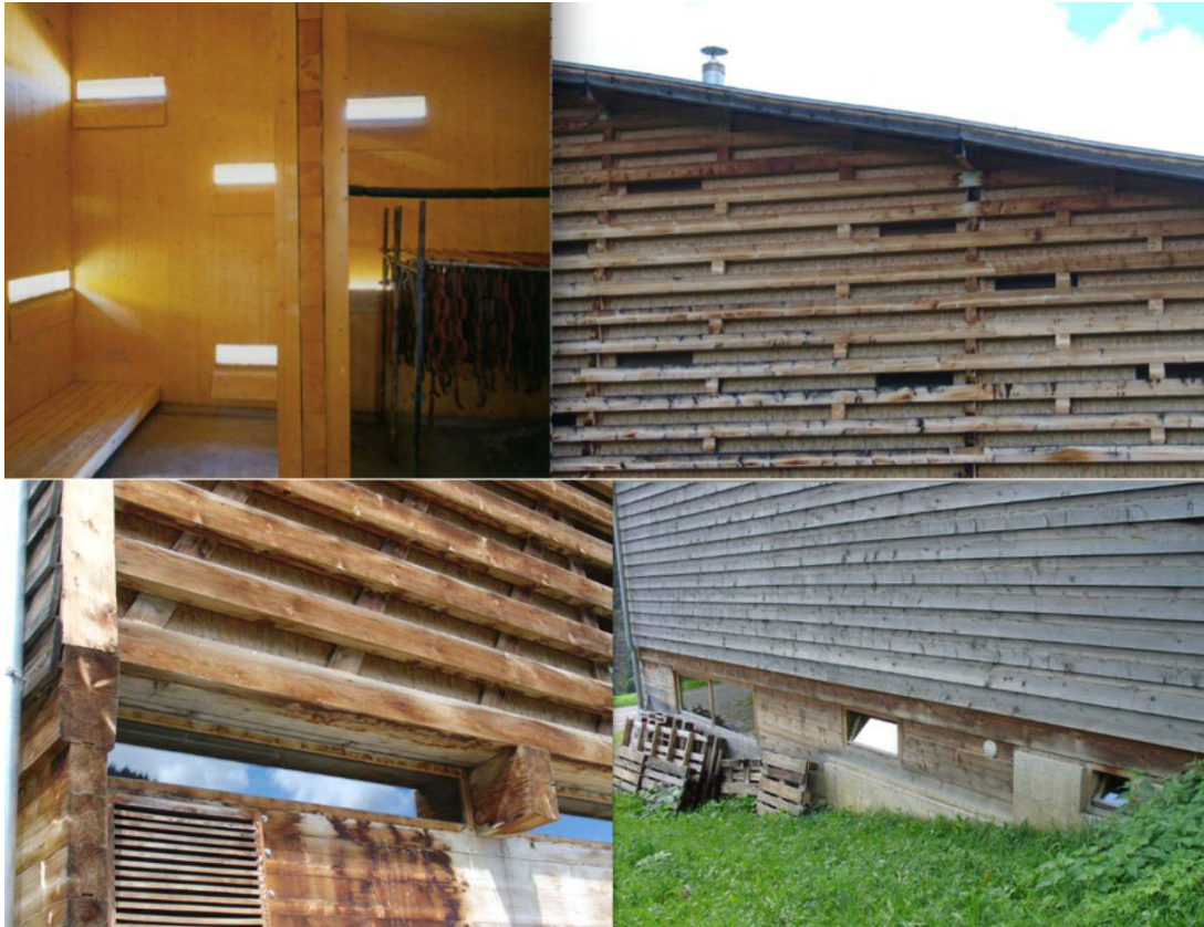
Figure 40: Design details. Upper left: adjustable vents in the upper floor of the cowsheds; upper right: vents from exterior; lower left: joint of timber; lower right: ventilation openings.
