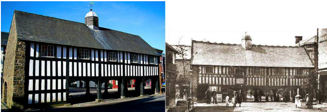
Figure 7: The well preserved timber framed market hall in Llanidloes in Wales, constructed in the 1610s (left: contemporary picture; right: historic image (Llanidloes Council, 2006))
