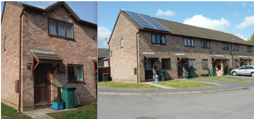
Figure 105: The front elevation of the house before (left) and after (right) retrofit (Forster and Heal, 2009)
