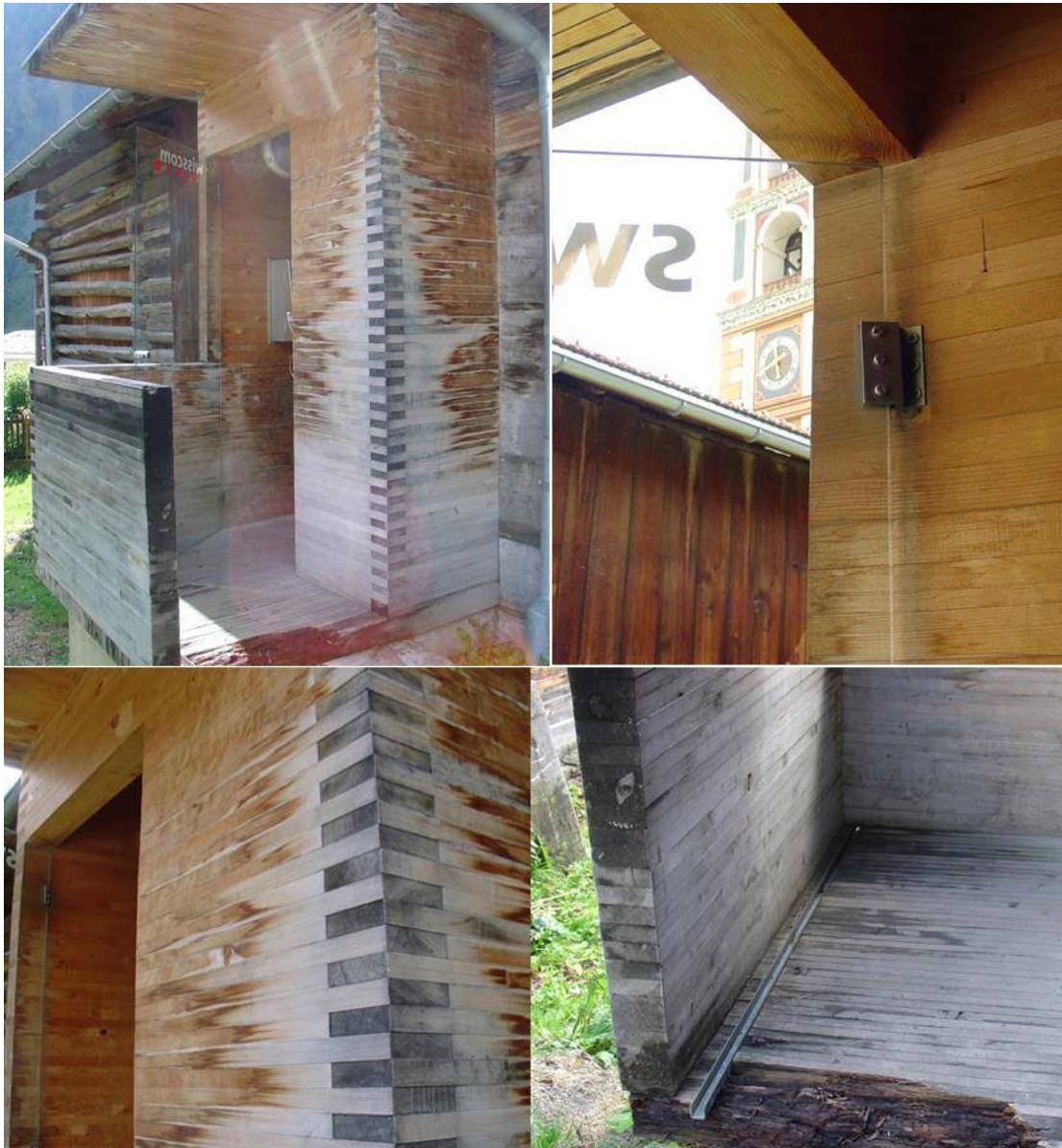
Figure 34: The telephone box in Vrin as found. Upper left: exterior; upper right: image of tower of St. Maria Church from the telephone box; lower left: corner joint of Strickbau using local timber; lower right: design detail
