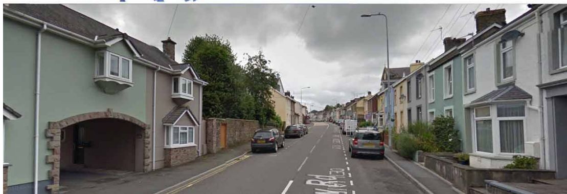
Figure 146: This image is to recall the final drawing at the end of Chapter 5 regarding the location of 4 designs and their roles to maintaining and enhancing the historic settlement. The lower image is the View of street frontage in New Road, which is the north boundary of Llandeilo conservation area.
