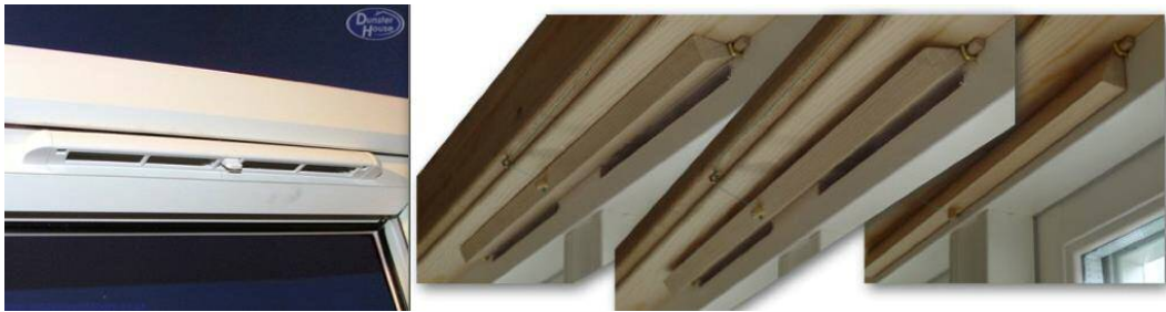
Figure 121: Window trickle vents made from plastic and timber
