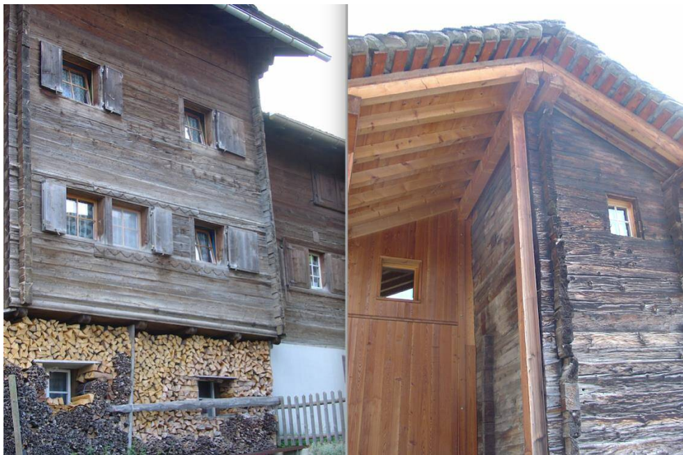
Figure 31: Domestic buildings in Vrin. Left: aged Strickbau building in use; right: aged Strickbau building with a new extension / restoration
