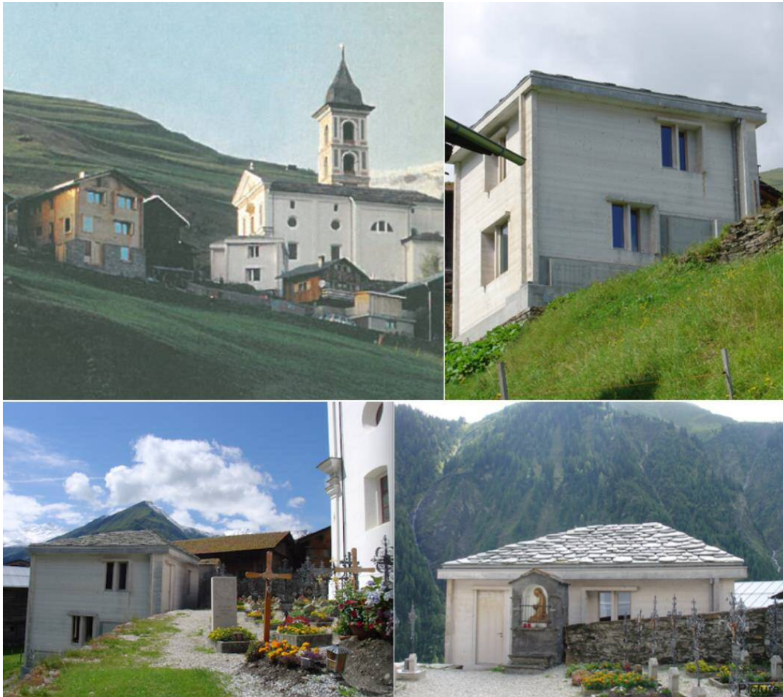
Figure 41: Mortuary for Vrin. Upper left: view of mortuary together with the church from the valley (Caminada 2008); Upper right: the mortuary; lower left: mortuary and cemetery; lower right: view of cemetery, mortuary, and valley from the church.
