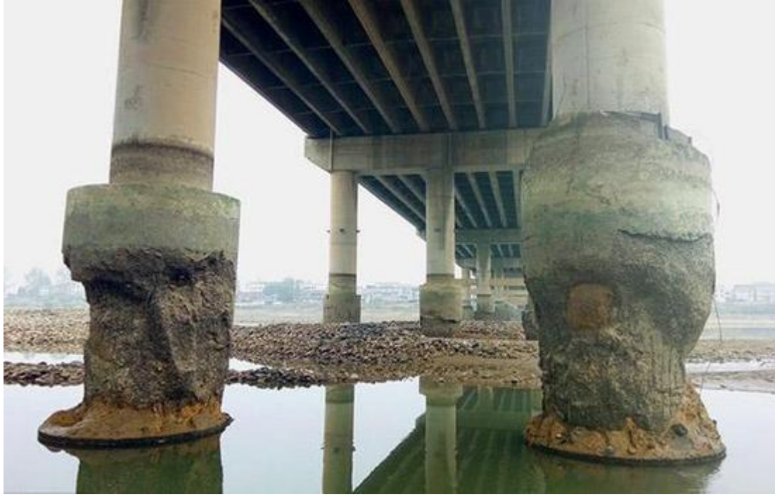
Figure.4 Voids and hungry spots on bridge piers (Voids on Lishui River Bridge, 2016)
