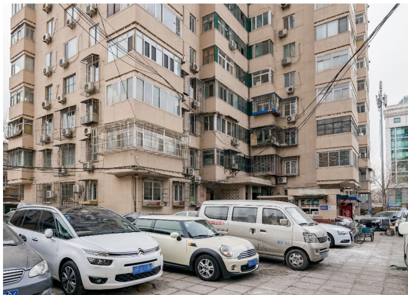
Figure 6.63 The building facade of Case 3 before the retrofitting
