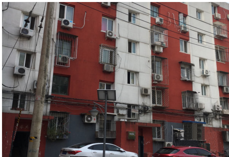
Figure 6.13 The building facade of Case 1 before the retrofitting
