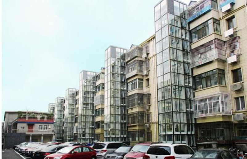
Figure 5.1 Elevator addition for existing residential building
