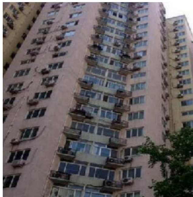
Figure 6.81 The building facade of Case 4 before the retrofit
