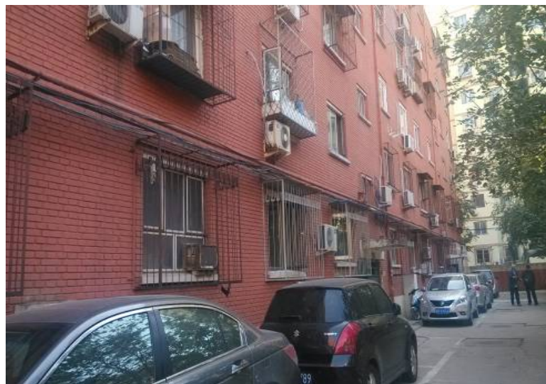
Figure 6.36 the building facade of Case 2 before retrofitting
